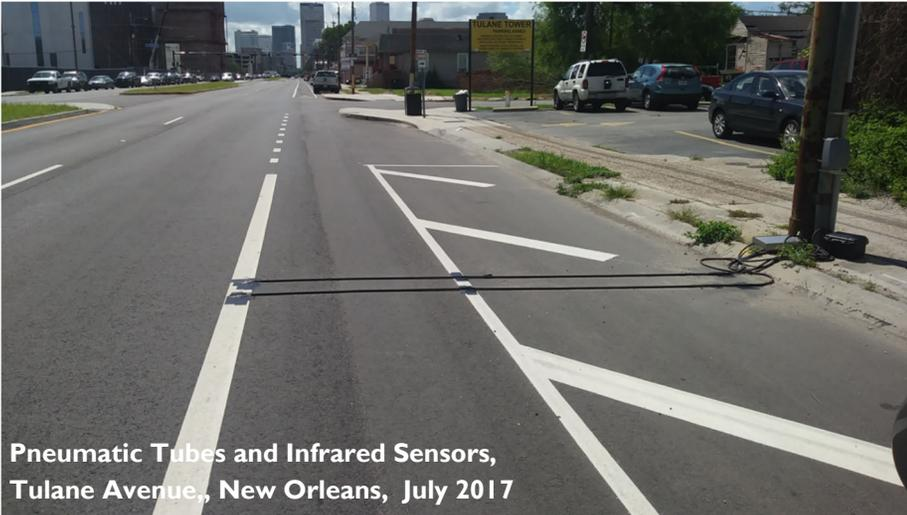
Pneumatic Tubes and Infrared Sensors,
